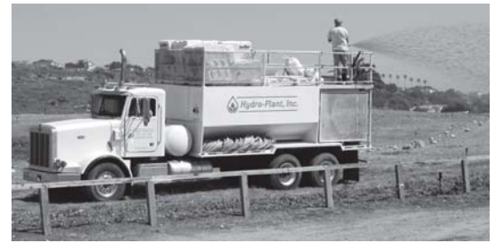
A mix of grass seed and mulch is sprayed onto the prepared ground.
